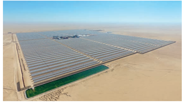
First stage of Al Sheqaya Renewable Energy Project, Kuwait. (Photo Source: GSSCPD).
